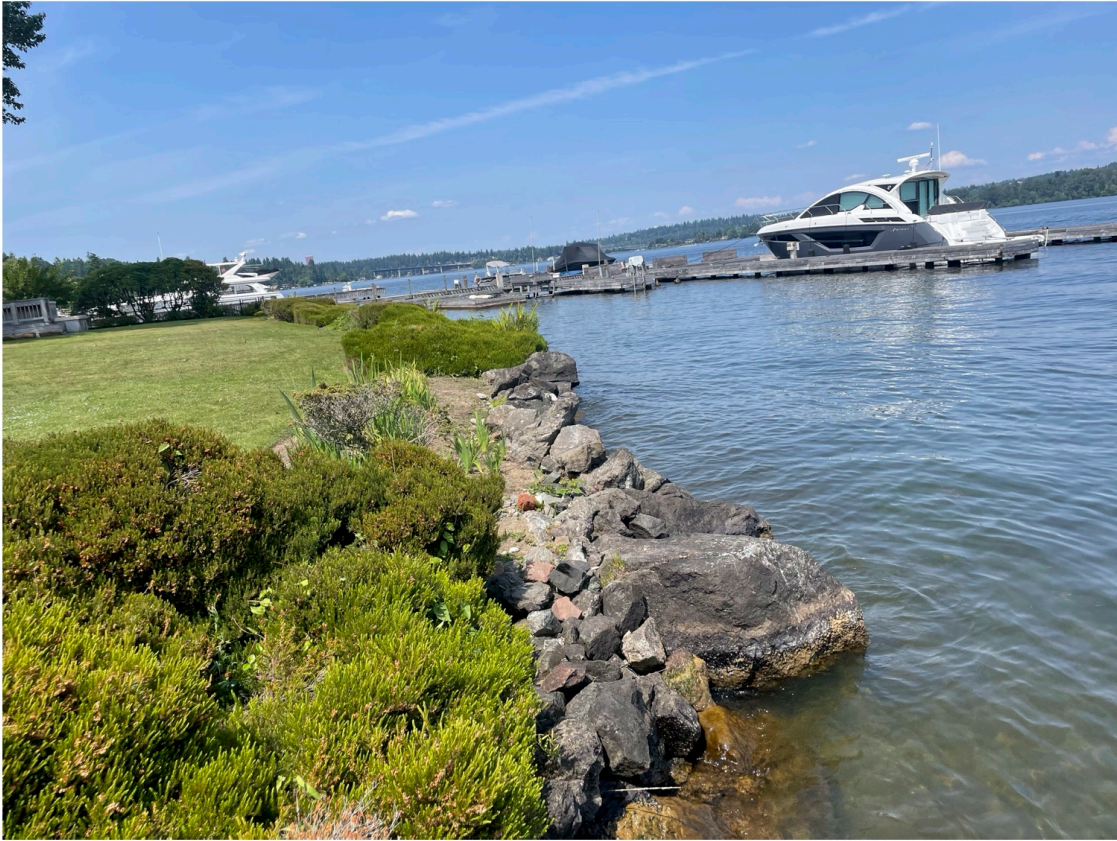
Photo 1 - Shoreline looking north from approximate area of new dock.
